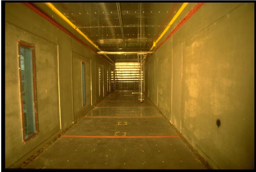
Interior of the tunnel
